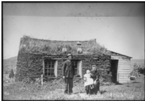
Figure 5: A sod roof in Milton, North Dakota, built by Ole Myrvik, a Norwegian Immigrant, c. 1896. Sod roofs were common in Norway because they added an additional layer of insulation and protection to the house. Norwegian immigrants brought the technique with them to the US and Canada.
