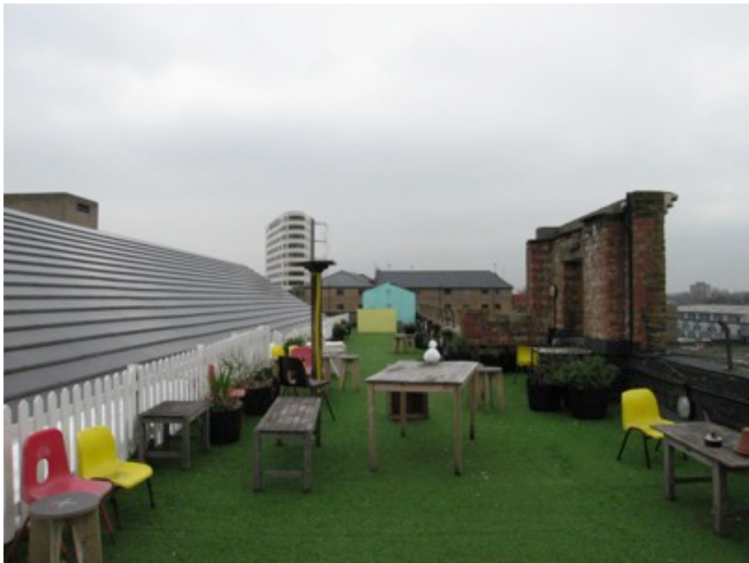
Figure 24: London's largest installation of PV panels (left), planters, and space for summer events such as film screenings and live music.
